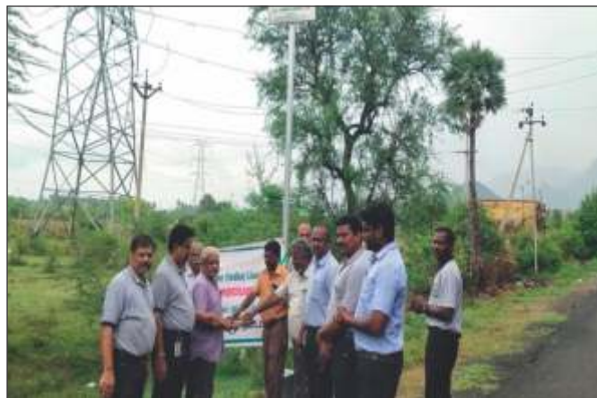
Solar Street Lamp installation
